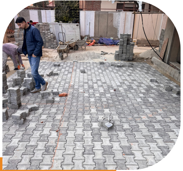
Fig : Pattern Laying
