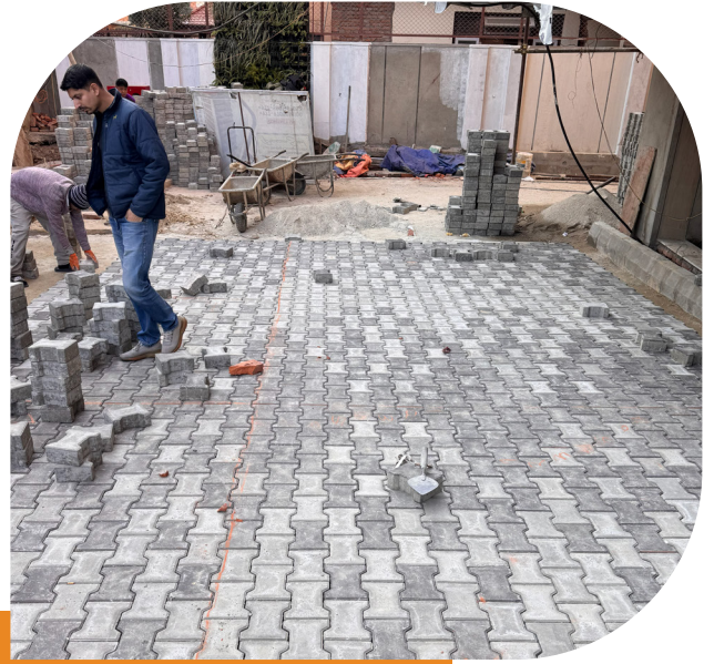
Fig : Pattern Laying
